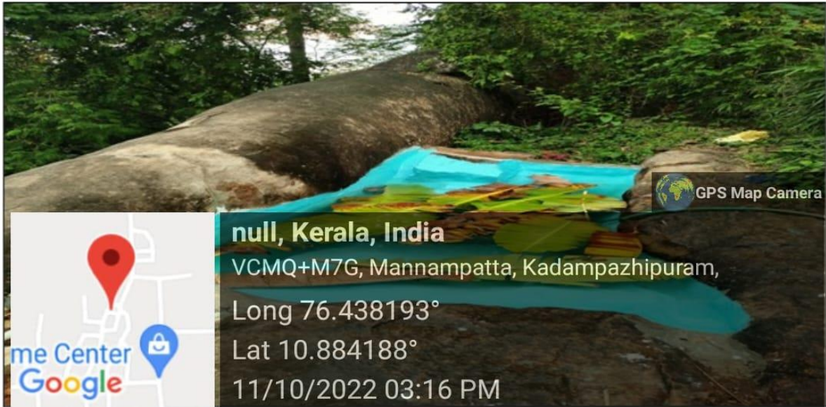
On 11/10/2022, banana leaves were placed in the water stored at Thamarakulam to absorb chemicals from cement and waterproofing.
