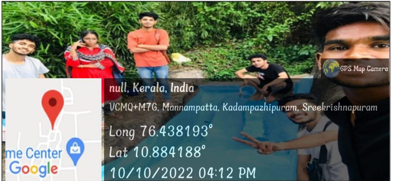
On 10/10/2022, Nature Club volunteers of VTBC completed the waterproofing work at Thamarakulam.
